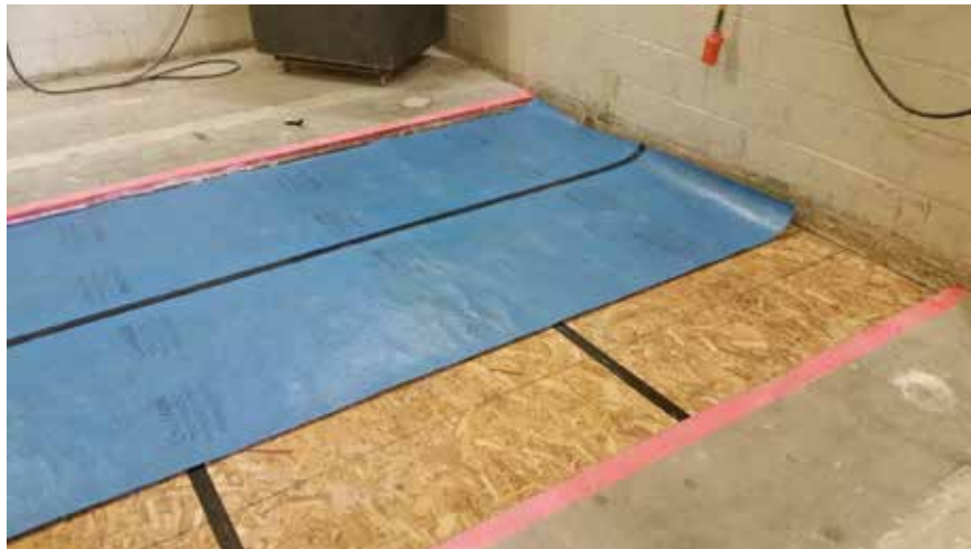
Figure 8 – Recycled cotton underlayment partially installed
