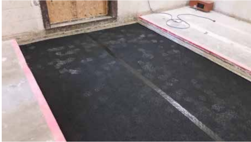
Figure 5 – Composite flooring layer 1 installed
