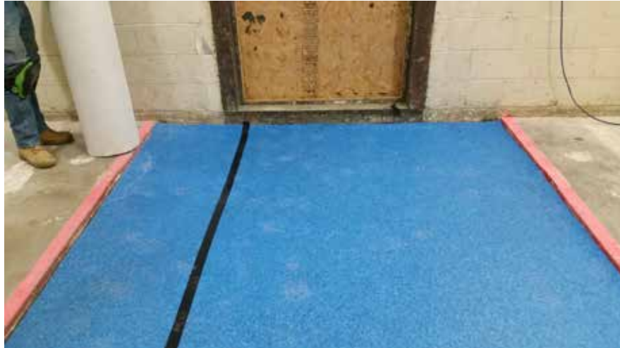
Figure 8 – Carpet pad installed
