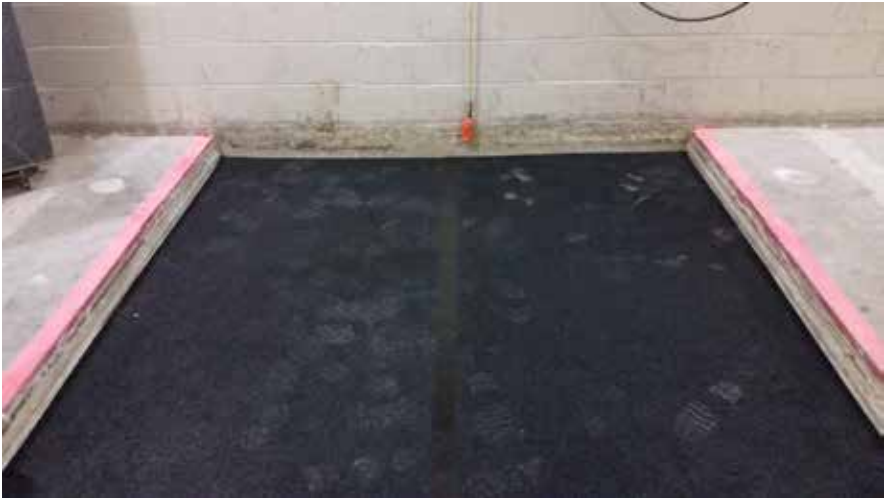
Figure 5– Composite flooring layer 1 installed over base slab
