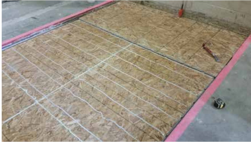
Figure 7 – Oriented strand board layers partially installed
