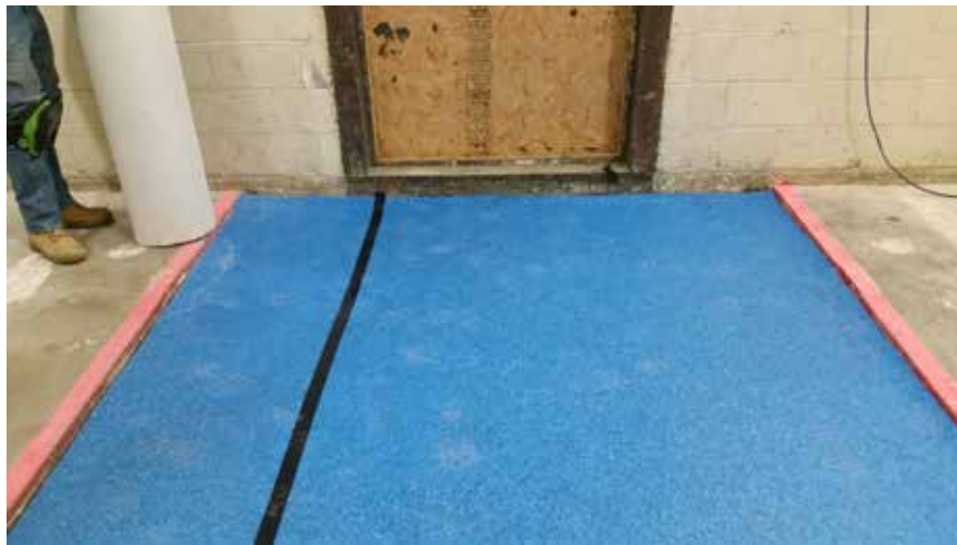
Figure 8 – Carpet pad installed
