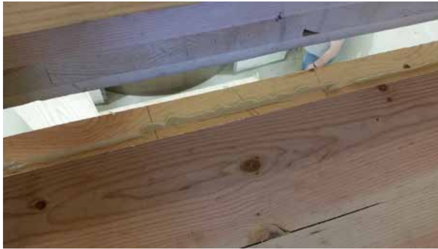
Figure 5 – Adhesive at shiplap joint
