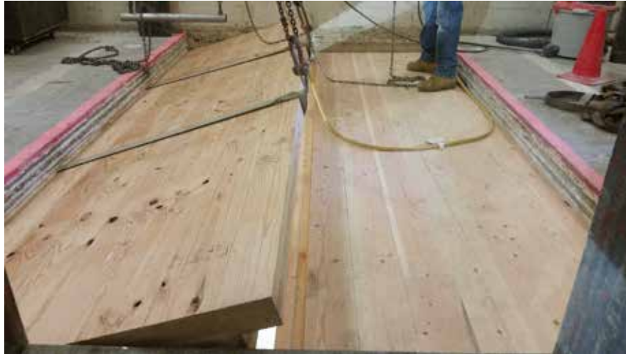
Figure 3 – Installation of cross-laminated timber base slab
