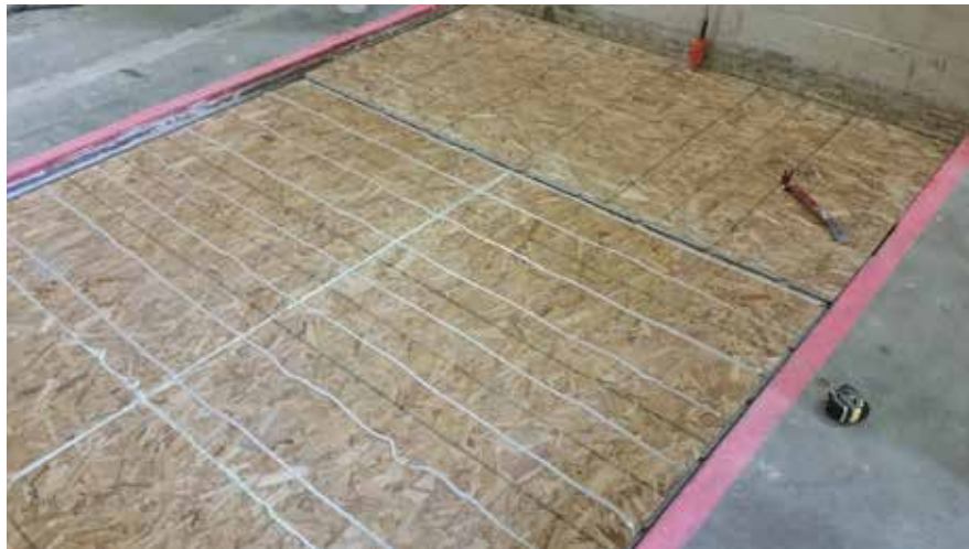
Figure 7 – Oriented strand board layers partially installed
