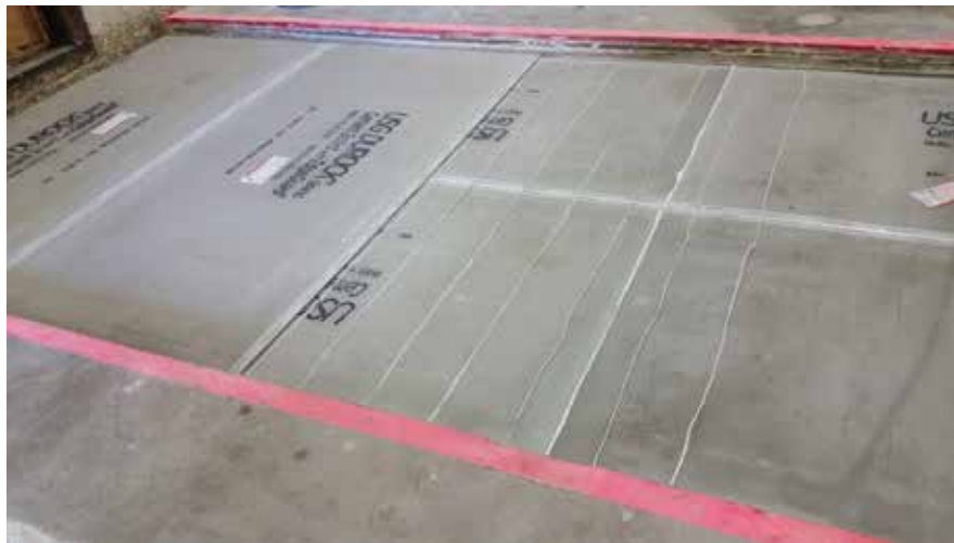
Figure 6 – Typical joint treatment and adhesive application pattern in cement board layers
