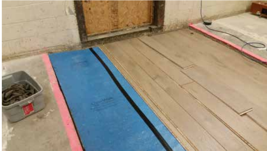
Figure 9 – Engineered wood flooring partially installed
