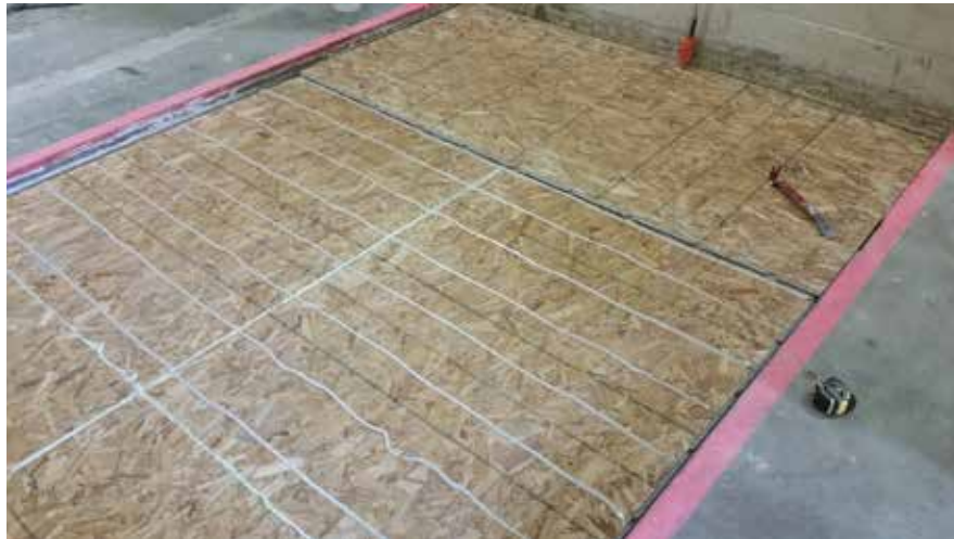
Figure 7 – Oriented strand board layers partially installed
