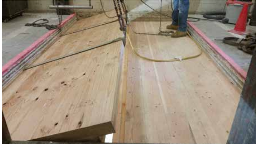
Figure 3 – Installation of cross-laminated timber base slab
