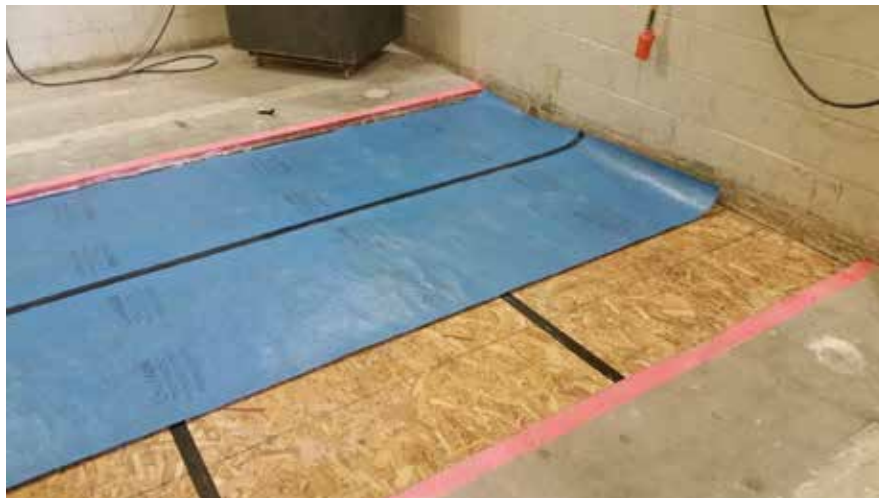
Figure 8 – Recycled cotton underlayment partially installed
