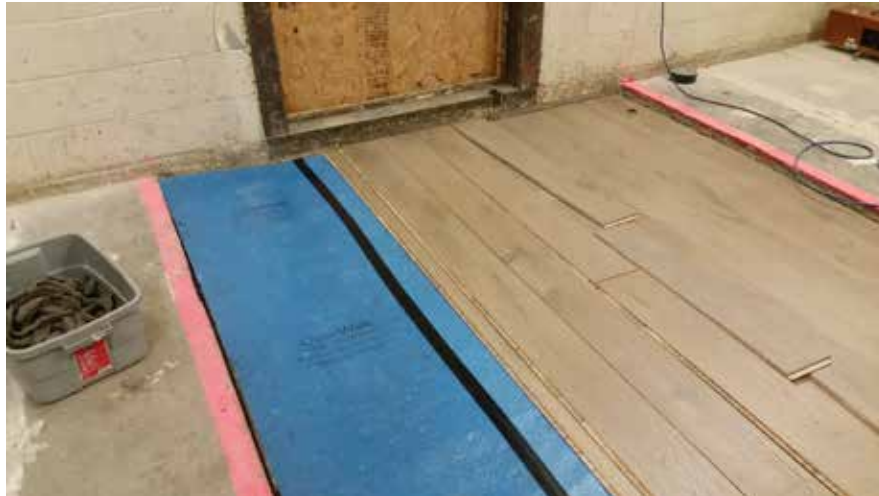
Figure 9 – Engineered wood flooring partially installed
