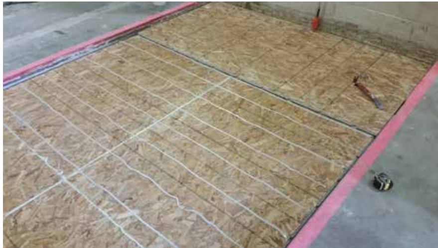
Figure 7 – Oriented strand board layers partially installed
