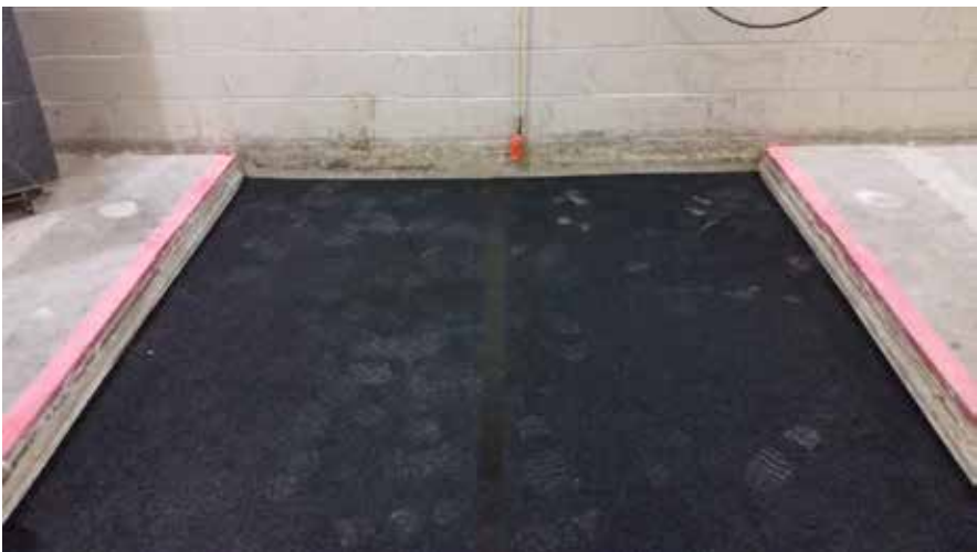
Figure 5– Composite flooring layer 1 installed over base slab
