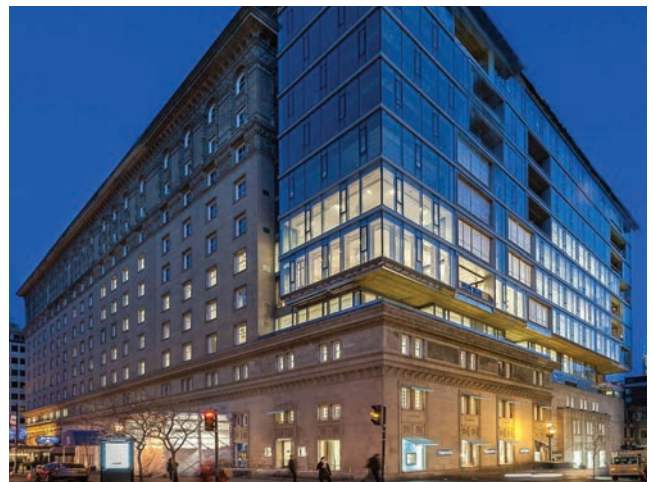
Picture 4. Ritz-Carlton Hotel, Montreal, Qc, Canada.
