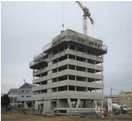
Picture 13. Example of a building with a concrete structure.
