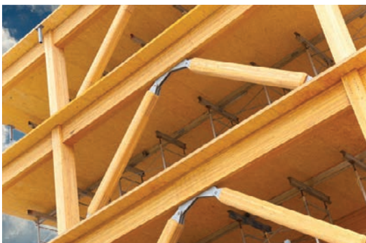
Picture 15. Example of a building with a Crossed Laminated Timber (CLT) structure. The University of British Columbia Earth Sciences Building . Architects: Perkins+Will Canada Architects Co. Picture by K. K. Law.
