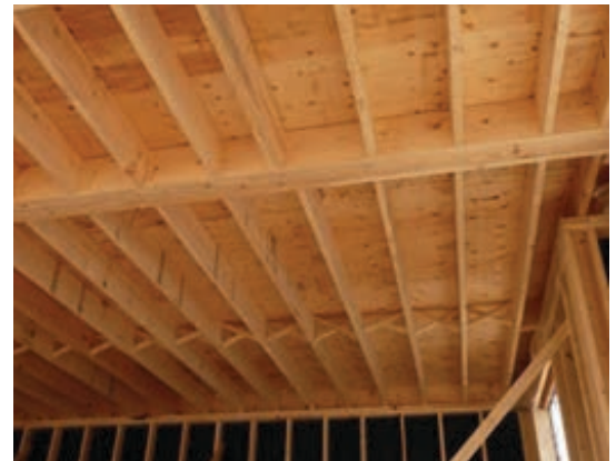
Picture 14. Example of a building with a timber frame structure.
