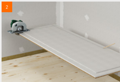
2 Cut away the protruding seam for the first installed row
