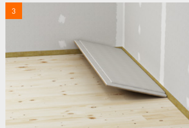
3 Lay fermacell® flooring elements
