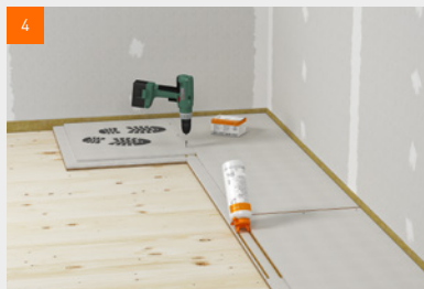
4 Apply fermacell™ floor glue seam area
