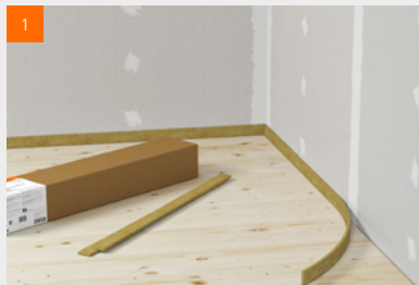
1 Install perimeter insulation strip, butt-jointed
