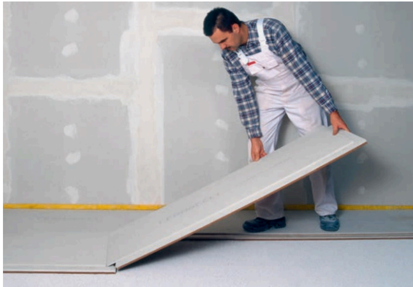
Figure 3 – Laying Fermacell Dry Screeds
